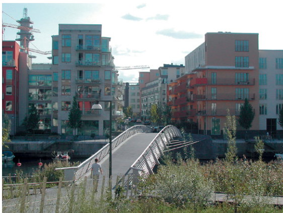
Figure 49 The Sickla bridge, constructed in duplex stainless steel.
