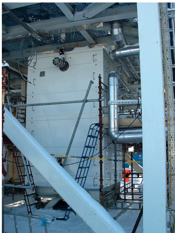
Figure 6 Composite fire-blast protection enclosure. Reproduced with permission from Solvent Composite Systems Ltd.
