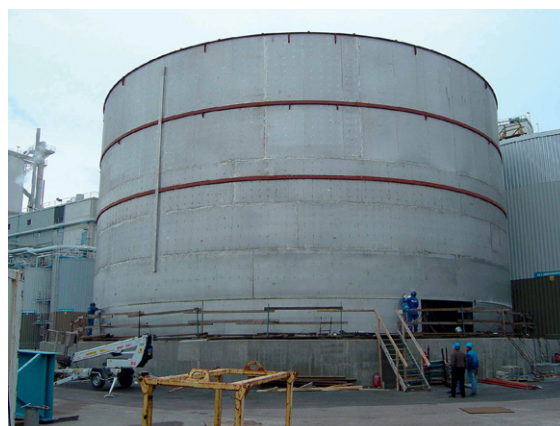
Figure 1 White liquor tank from the pulp and paper industry built in a recently developed stainless steel grade, S32101 (1.4162).
