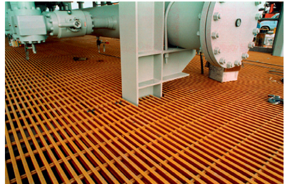
Figure 5 A glass-phenolic grating on the Mars Platform in the Gulf of Mexico, Courtesy of Strongwell.
