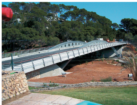
Figure 52 Bridge constructed in stainless steel, located at Menorca.
