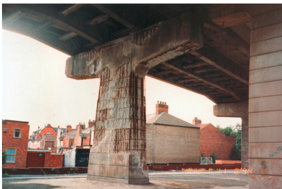
Figure 3 Chloride-induced corrosion.
